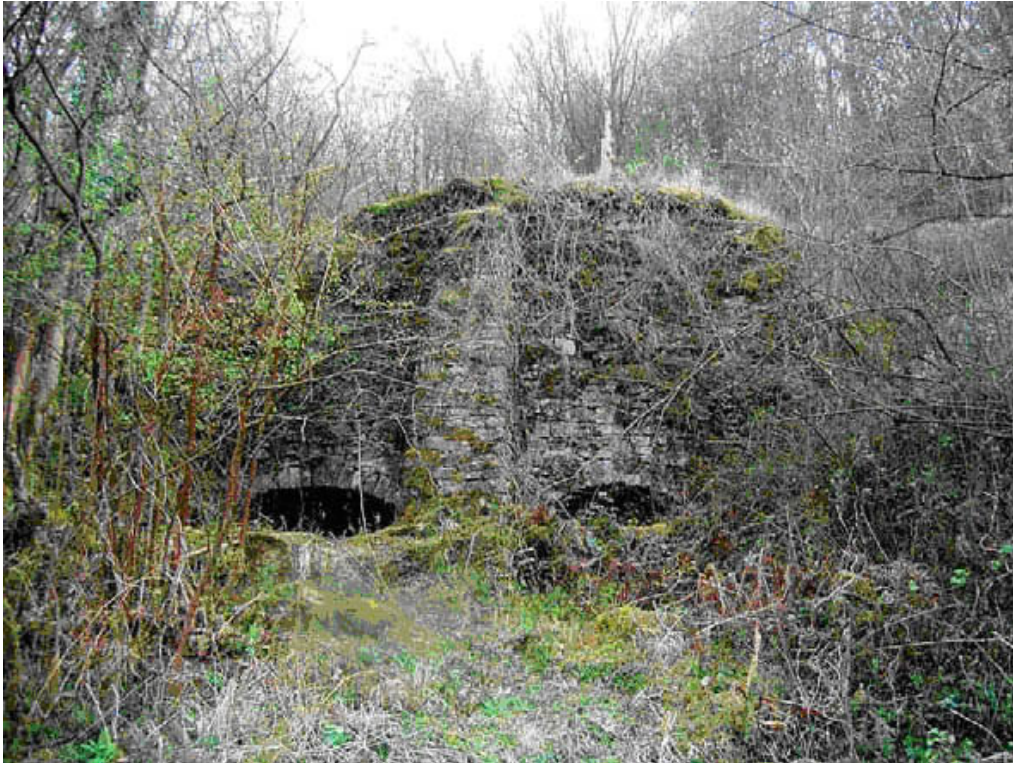
The Coppett Hill Lime Kiln before and after restoration
